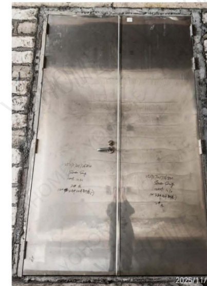
Exposed Side Prior to the Fire Test
