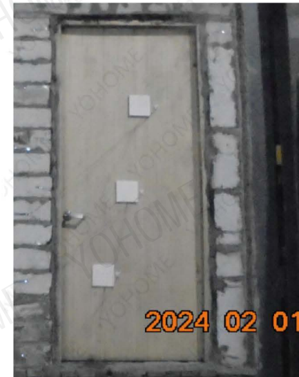
Photo No. 4 Unexposed Side after 40 Minutes
