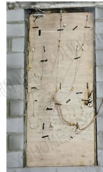
Fig. 5 Unexposed Side after 60 Minutes of the Fire Test 1
