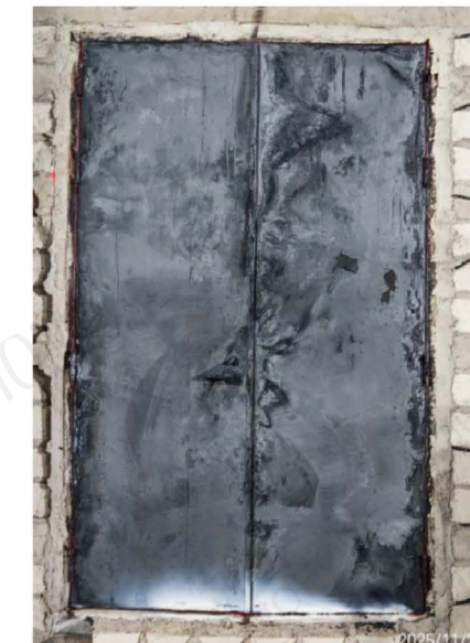
Exposed Side after the Fire Test
