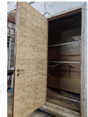
Fig. 16 Exposed Side of test door assembly after air leakage test 4
