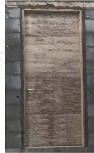
Fig. 1 Exposed Side Prior to the Fire Test 1
