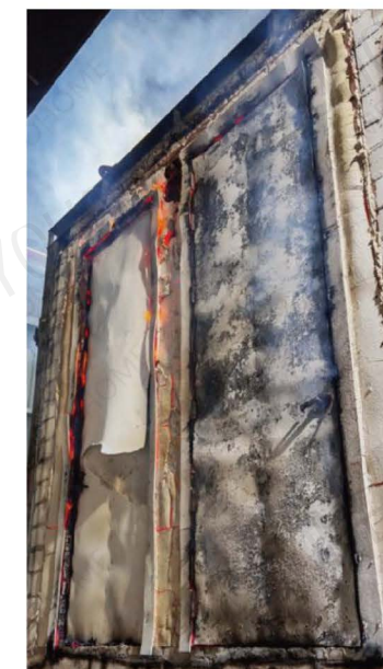
Photo 8 - Exposed Side after 90 Minute
