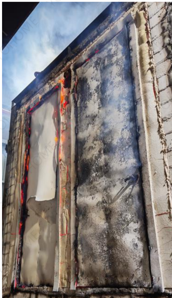
Photo 8 - Exposed Side after 90 Minutes
