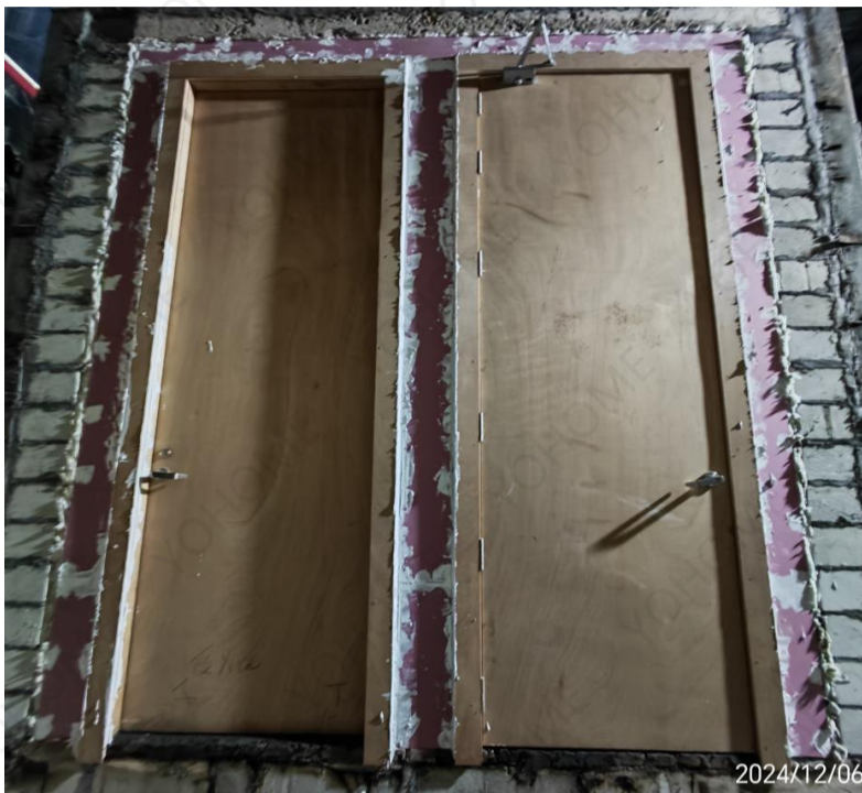
Photo 1 – Exposed Side Prior to the Fire Test
