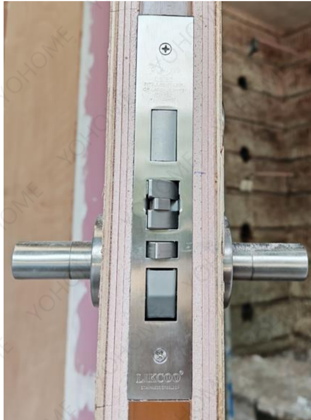
Photo 3 – Latching Mechanism
