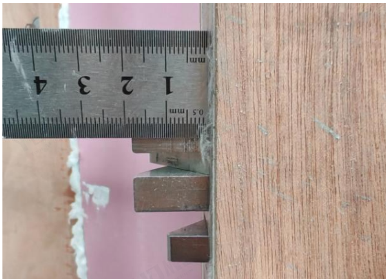
Photo 3 – The Latching Mechanism
