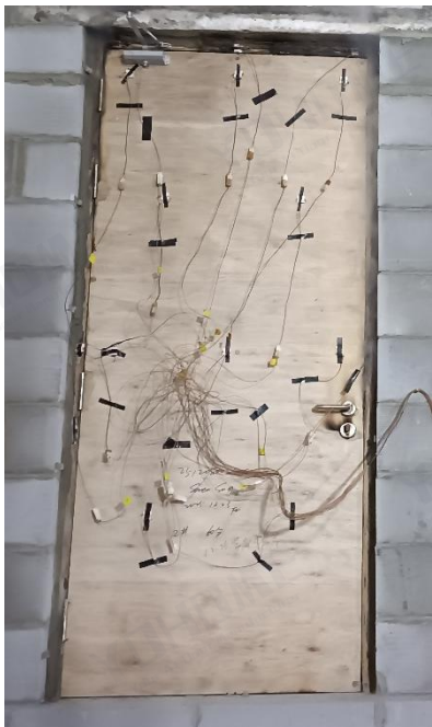
Fig. 4 Unexposed Side after 40 Minutes of the Fire Test 1
