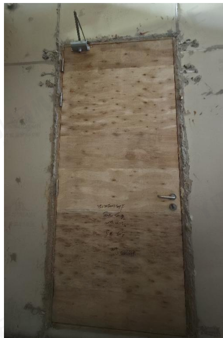
Fig. 20 Exposed Side of test door assembly after air leakage test 5
