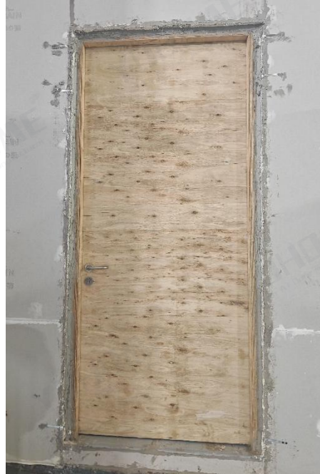
Fig. 19 Unexposed Side of test door assembly after air leakage test 5
