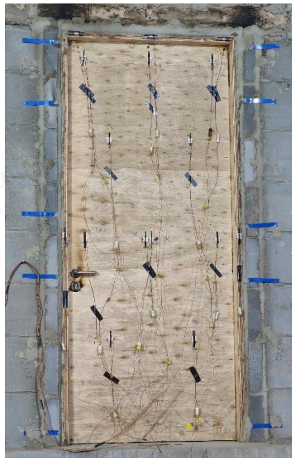
Fig. 10 Unexposed Side after 40 Minutes of the Fire Test 2
