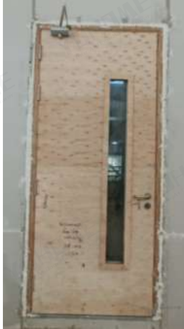
Fig. 7 Unexposed Side of test door assembly before air leakage test 2
