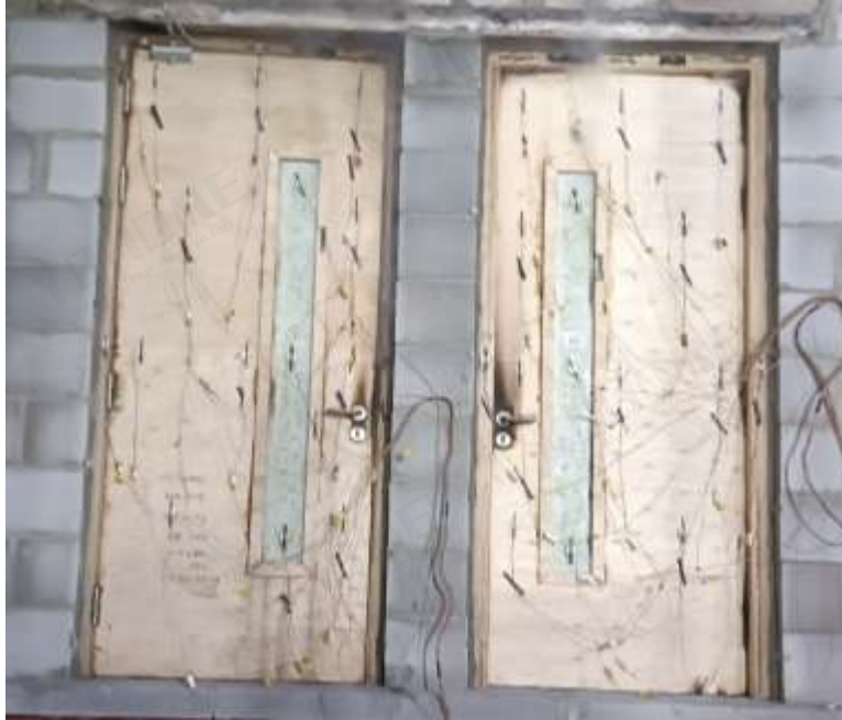
Fig. 5 Unexposed Side after 102 Minutes of the Fire Test 1
