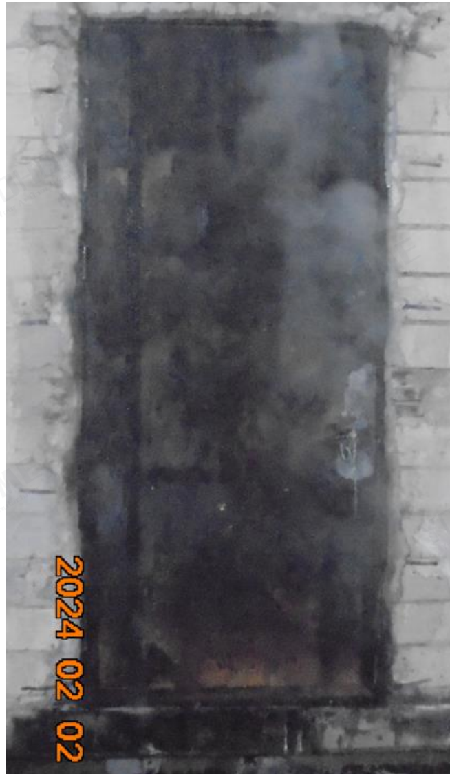
Photo No. 7 Exposed Side after Hose Stream Test
