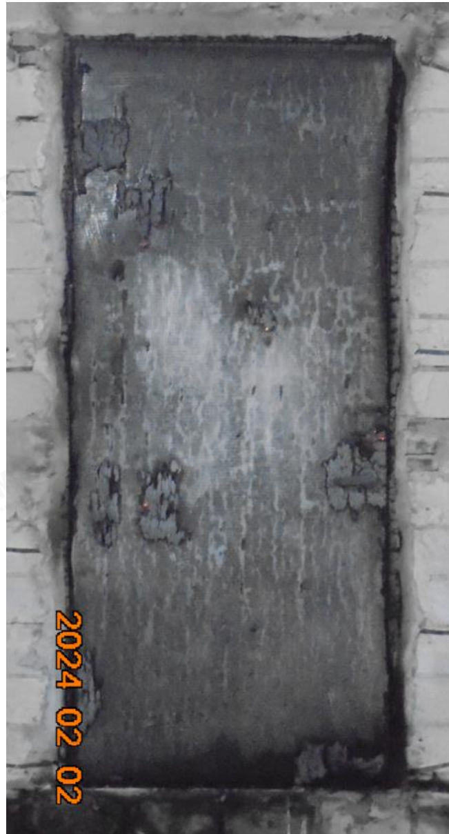
Photo No. 5 Exposed Side after 20 Minutes
