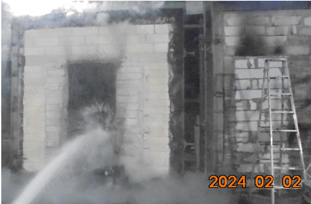
Photo No. 6 Exposed Side during Hose Stream Test
