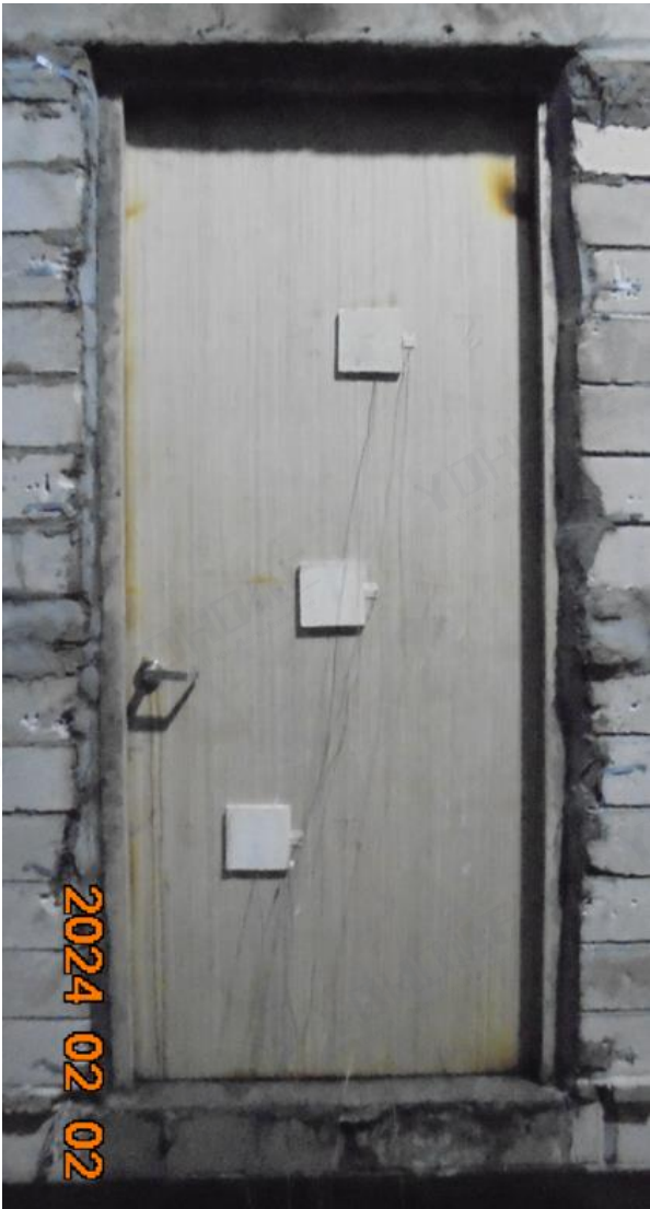
Photo No. 8 Unexposed Side after Hose Stream Test
