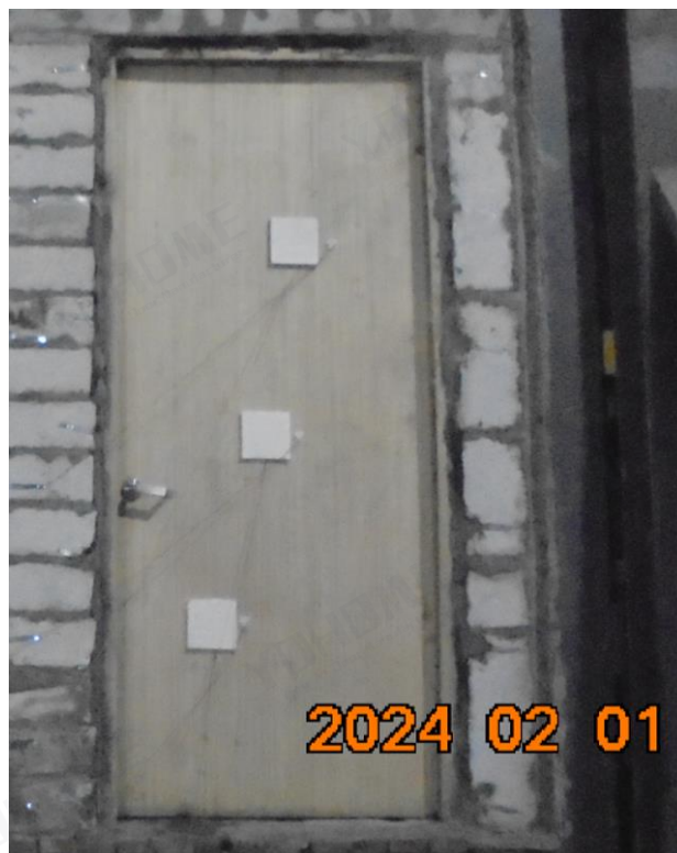
Photo No. 4 Unexposed Side after 40 Minutes
