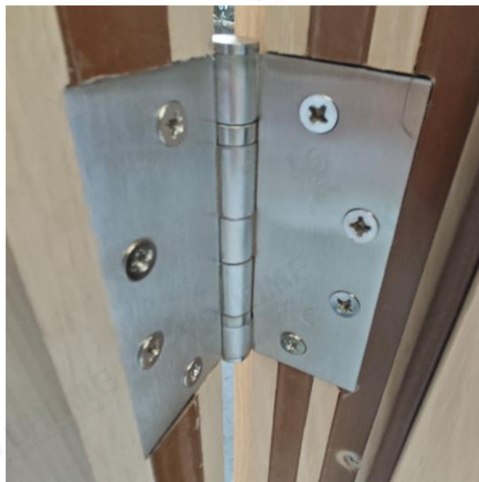
Photo 4 – Hinge and Intumescent Strip
