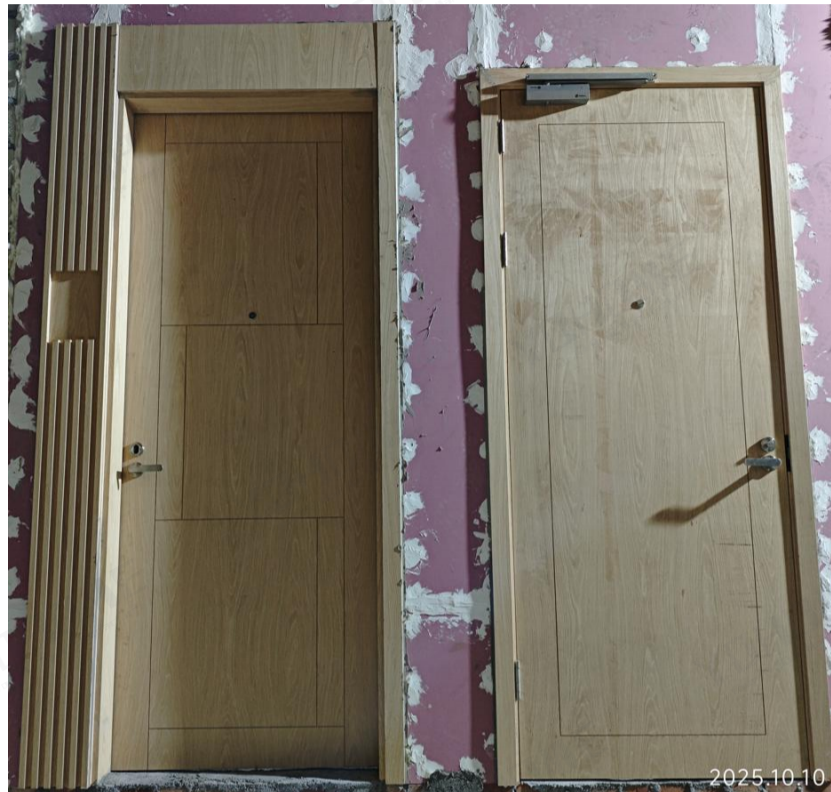
Photo 1 – Exposed Side Prior to the Fire Test
