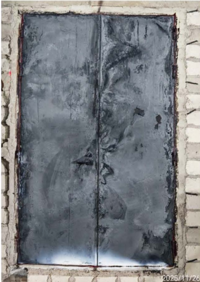
Exposed Side after the Fire Test
