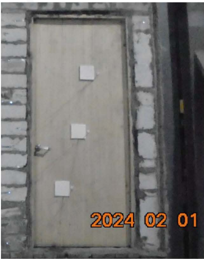
Photo No. 4 Unexposed Side after 40 Minutes
