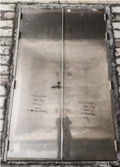
Exposed Side Prior to the Fire Test
